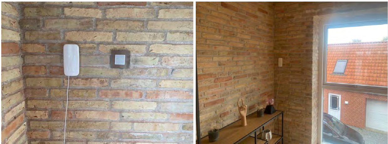
Figure 60: Left picture: IC-meter in the kitchen next to Niko Multisensor. Right picture: IC-meter in Small living room.
