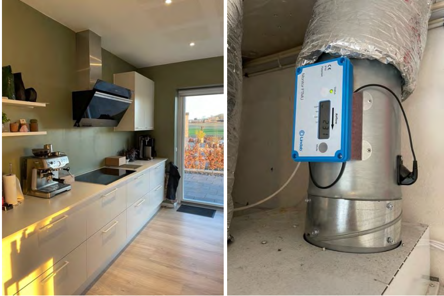
Figure 9: Left picture: Cooker hood in the kitchen. Right picture: Air flow sensor Lindab UltraLink FTMU.
