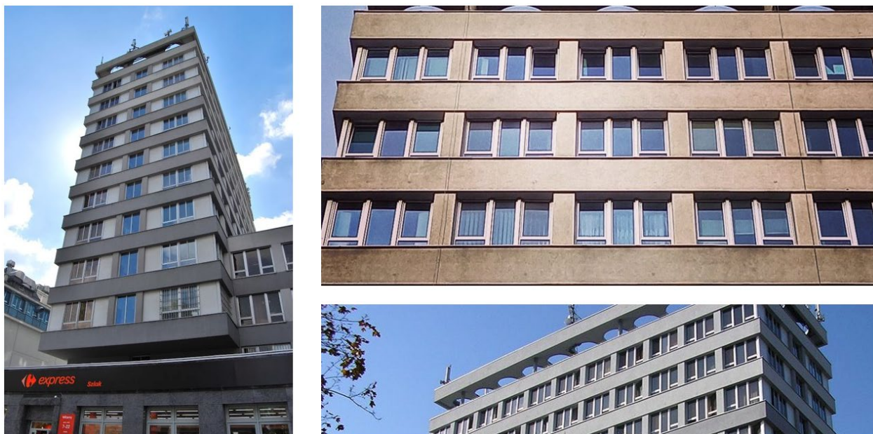
Figure 1 Photos of the building
