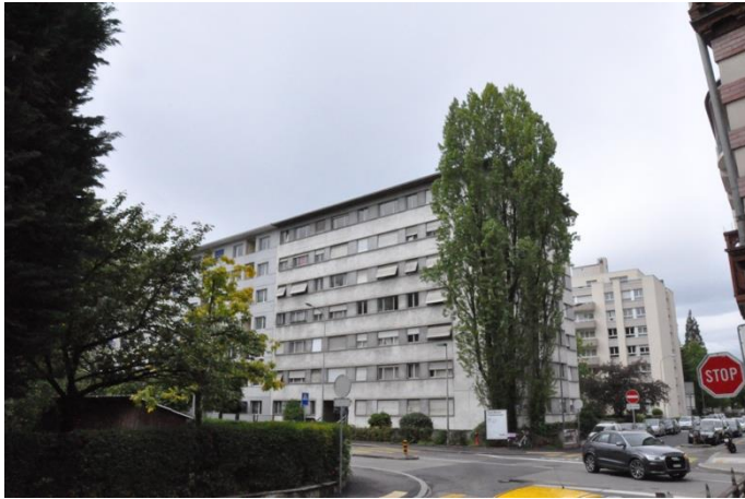
Figure 1: Wendt 35 before its refurbishment
