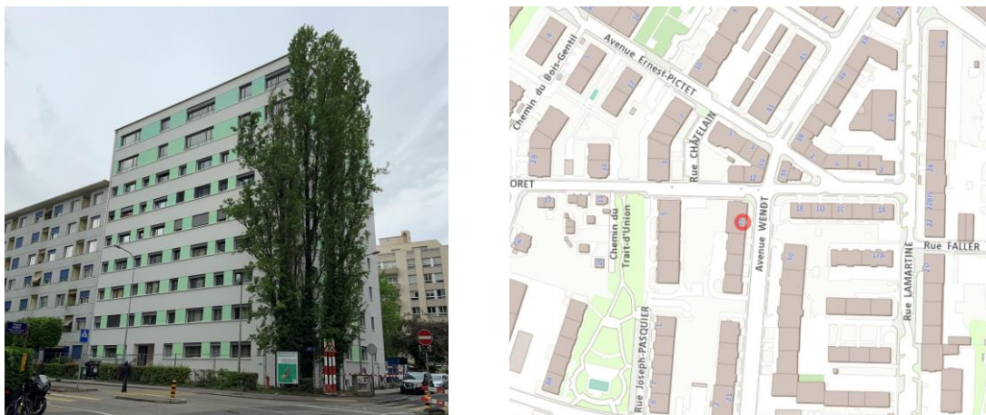
Figure 2: On the left: Picture of the south-eastern façade. On the right : Cadastral plan of the Wendt avenue
