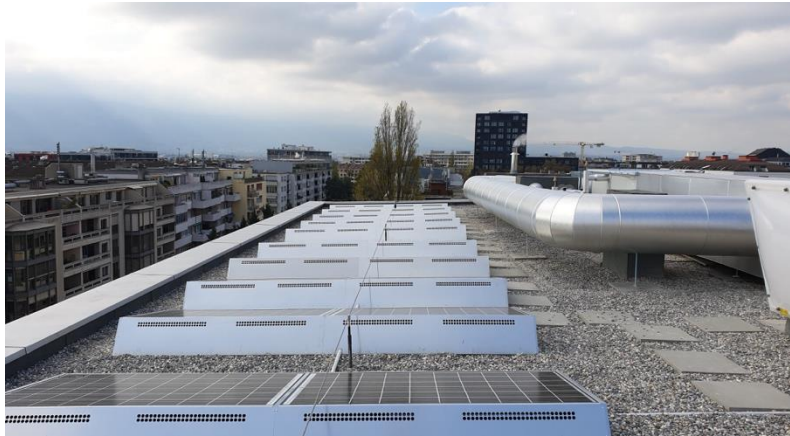
Figure 7: Picture of the roof. The available space is shared between the ventilation extraction and the PV panels.
