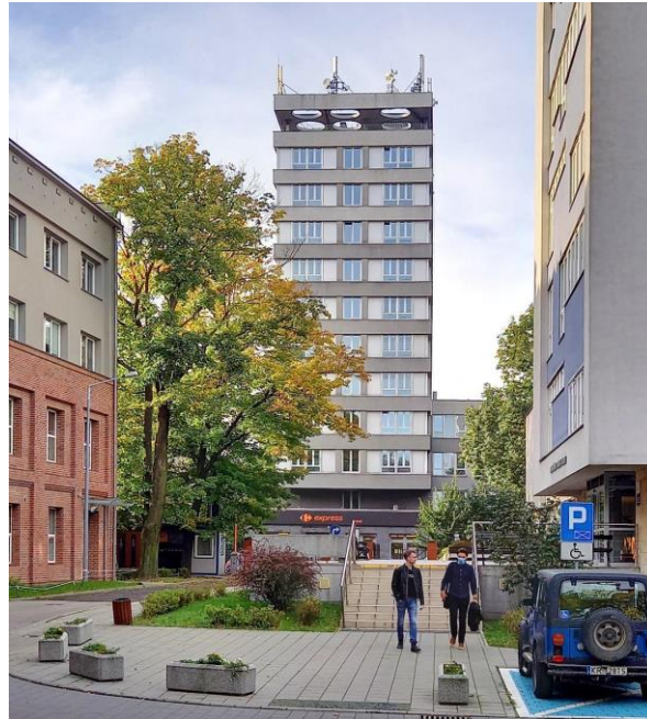
Figure 18: Building demonstration case in Krakow
